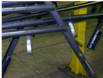
Tags hanging from stair system parts during production
