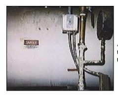
Asbestos pipe and boiler insulation does not present a hazard unless the protective canvas covering is cut or damaged in such a way that the asbestos underneath is actually exposed to the air.
