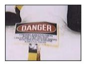
Pipe and boiler insulation that contains asbestos will be labeled with identifying stickers and placards.
